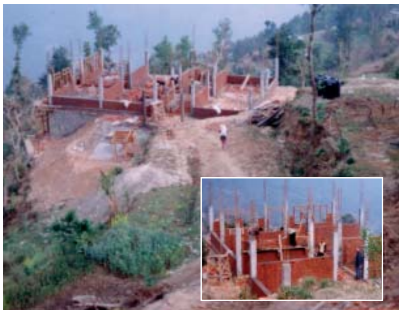
Building of the Bhattidanda School is now underway
